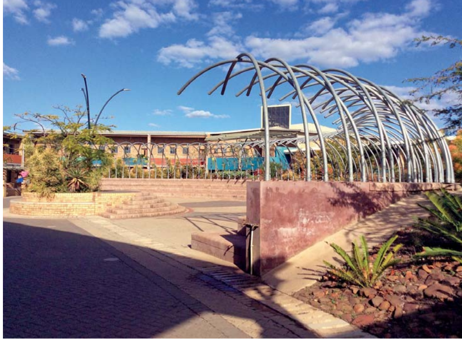
ABOVE: View across the Ngqukane to the library in the southern corner. The thermal chimney is placed over the media centre to encourage cooling by way of convection currents.
