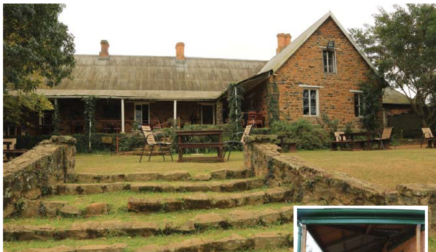
INSET: The veranda of Yarrow in the Karkloof, 1860, a structure supported on sneezewood posts and the shale stone wall.
