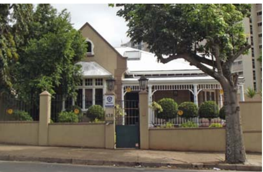
ABOVE: 438 Clark Rd, Durban. Houses for Mr WS Cornelius Esqre (sic), Clark Rd, Durban, by architect JJH Lübke, 1912. Note that in realisation the house was inverted from the plan.
