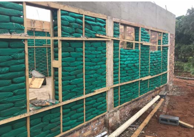
ABOVE: Sandbagged construction. RIGHT: Drone view of excavated foundations.
