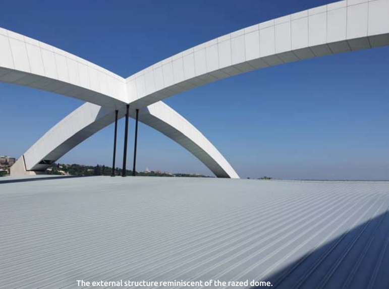
The external structure reminiscent of the razed dome.
