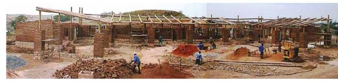
Mud bricks on a concrete block plinth; hollow piers attached and detached support the roof structure of gumpoles.
