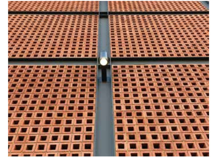
Detail of the perforated screen filling the steel frame.
