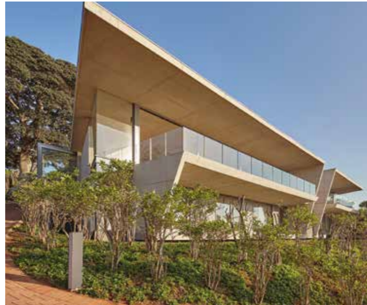
Apartment A from south-east. Note the frame at left to allow the sliding doors to open fully.
