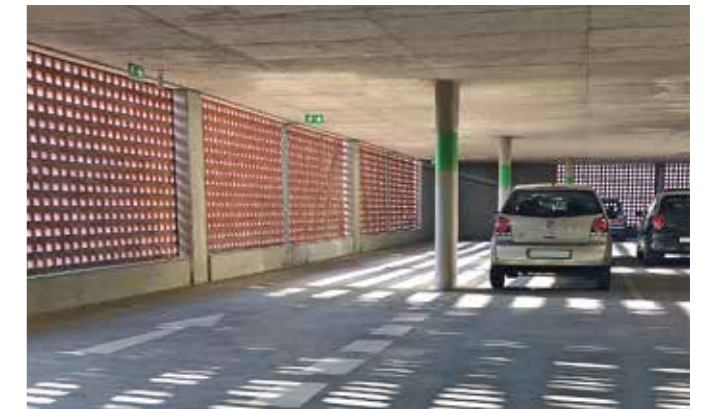
Interior of a parking level.
