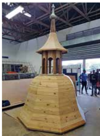
Timber structure awaiting lead covering.
