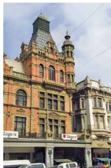
The oriel turret at right, with its roofs repaired and re-leaded.
