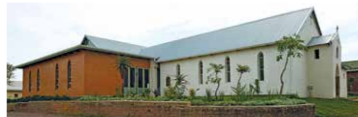
View from south, with old at right, extension at left.
