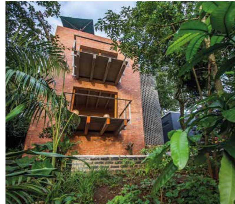
View from south-east.
