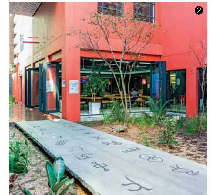
The functional need for a hardened path to cross the courtyard and, effectively, unite the campus of Regent Business School, saw Andries Botha being commissioned with a creative intervention. The 'bridge' which he conceived, and was completed in January 2017, contains selected symbols or pictograms by which earlier civilisations communicated, sand-blasted into the granite floor slabs. This communication means is not dissimilar from today's use of emoji, and serves to affirm that past and present are a continuum, the foundation on which an academic institution is built. See also The lost language walk(a)way published by Architects Collaborative cc, 2018.
