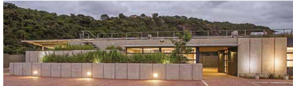
Well greened north elevation.
