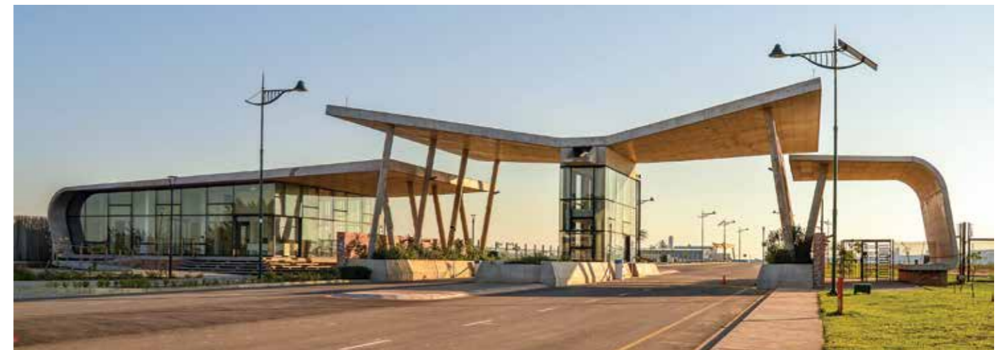
View of RBIDZ gateway from the east.
