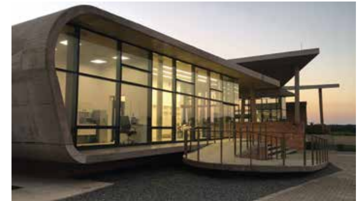
View from south-east with ramp at right.
