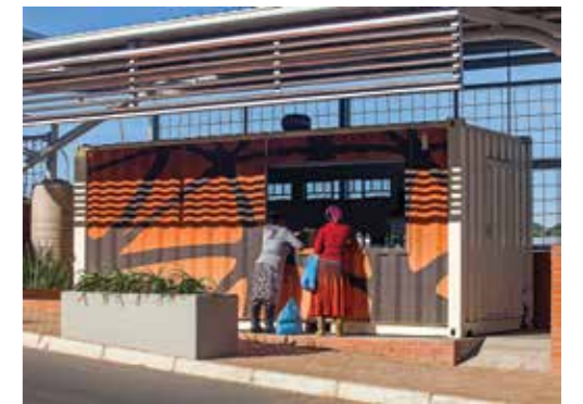
Detail view of one trader container in use.
