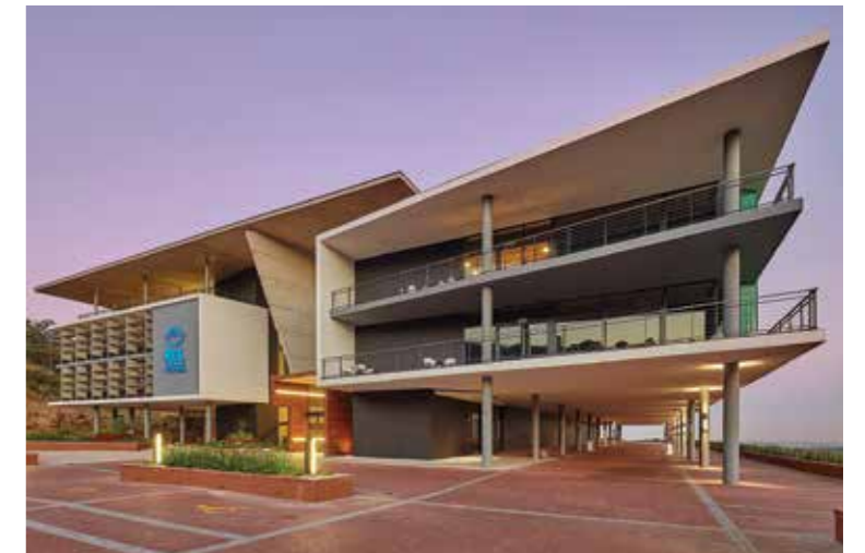
The office component on the podium.
