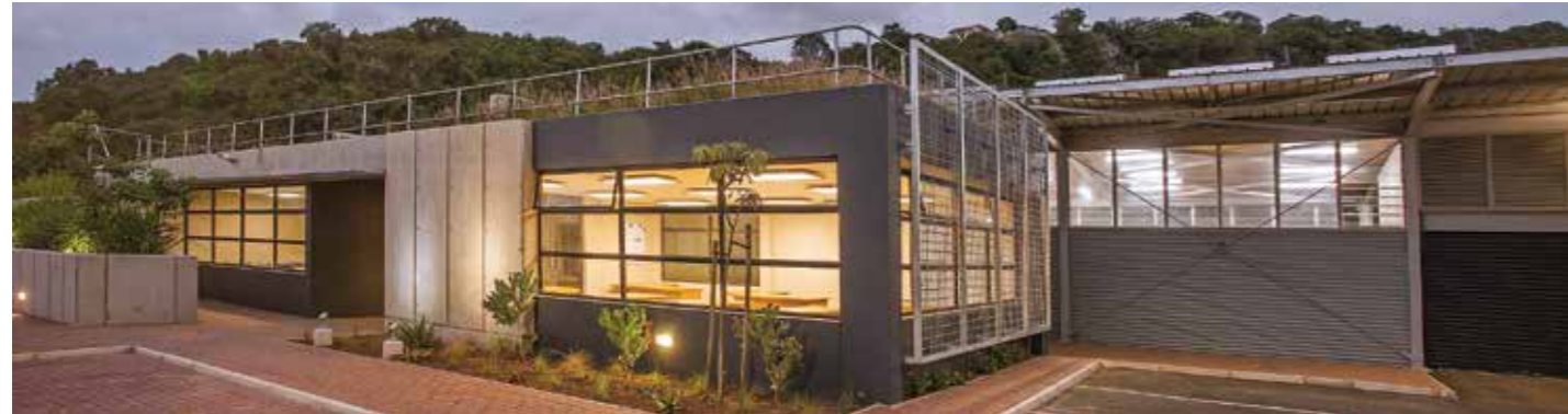
Administrative component from north-west.
