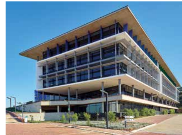
Articulation of the south-east with horizontal baffles and widely spaced angled fins. This façade acknowledges the orthogonal exterior of the adjacent building, Westside office park, which landed for its architects, Jay & Nel, a Special Mention in 2013 (see KZNIA Journal 2/2013).
