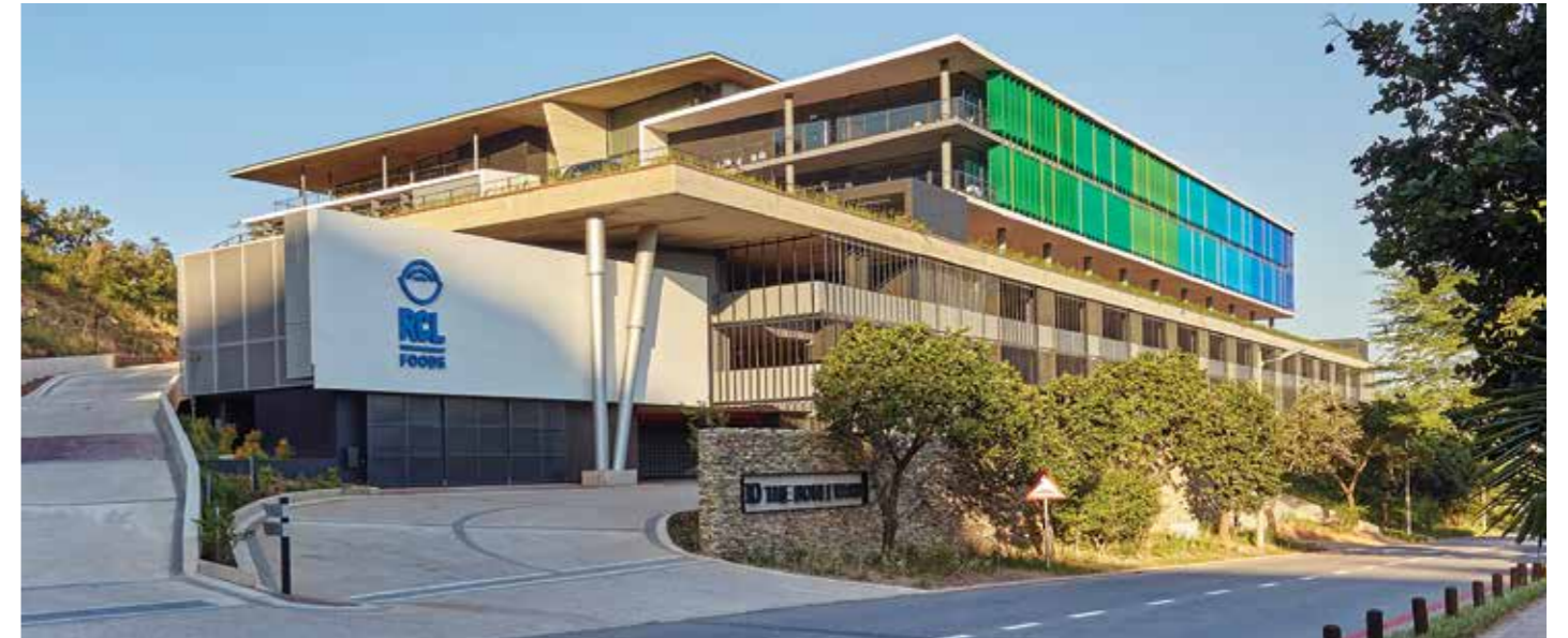
The building from north-west within the constricted site on The Boulevard, with office component articulated from the parking levels. Note the closely spaced fins on the office floors to mitigate the influence of the west sun, and the colouring thereof from the blue on the end towards the ocean (right) to the green on the inland (left).
