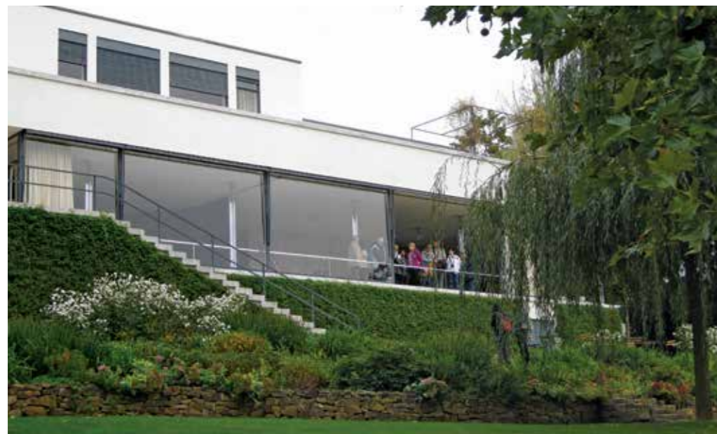
South elevation where a group was admiring the open portion of the glass wall, as the large format pane of glass had been lowered to convert the lounge into a belvedere or veranda.
