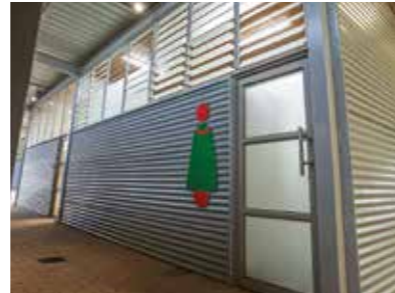
Communal facilities of light-weight construction.
