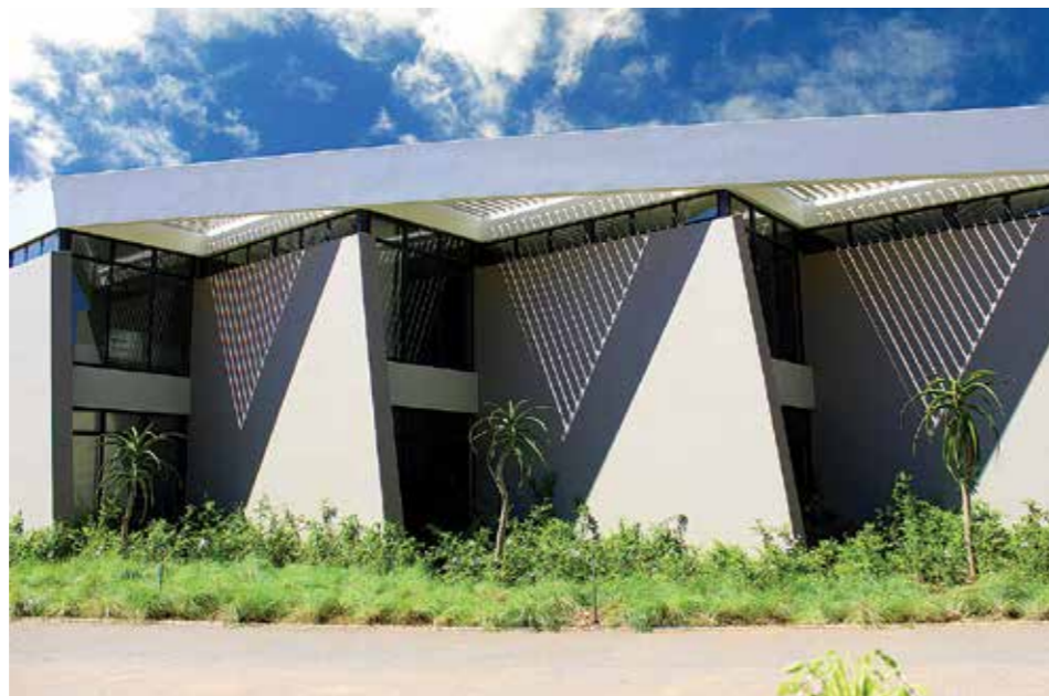
Headquarters for Earthworks, Romead Business Park, Pinetown
