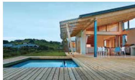
House Levinson, Simbithi Eco-Estate, Ballito
