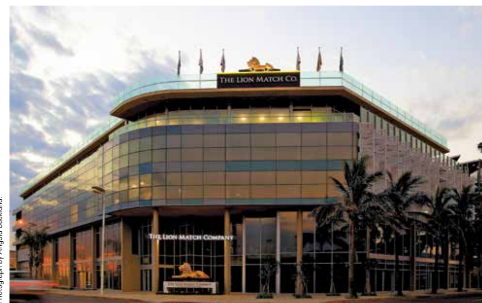
Lion Match Head Office and Distribution Centre, Point
