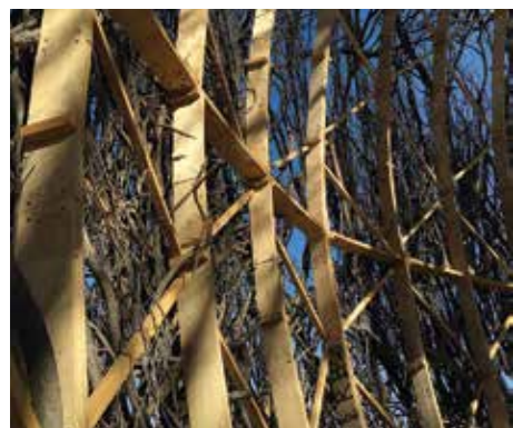
Detail of dome structure
