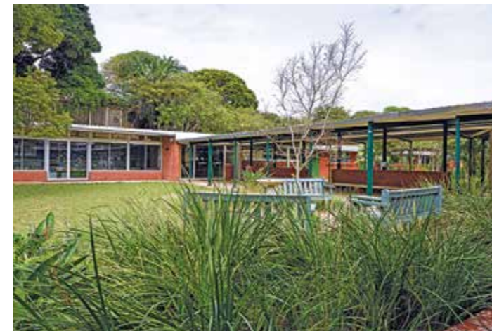
10. Junior After Care (left) and 11 New Covered Walkway (right)
