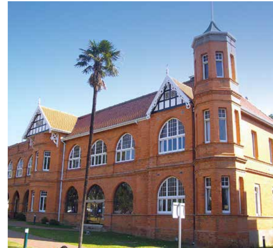
East wing in which the lower veranda arcading was surreptitiously enclosed with security glazing
