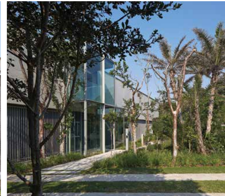
Entrance on lower ground floor
