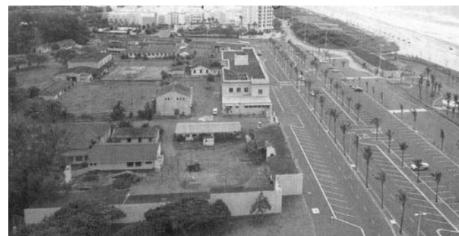
10. Aerial view from the south, 2011, before demolition of secondary structures.
