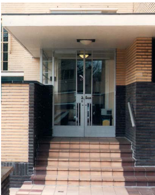
ABOVE: The buff paving of the staircase in the width of the steel-framed doors, under the cantilevering flat roof of a side entrance.
