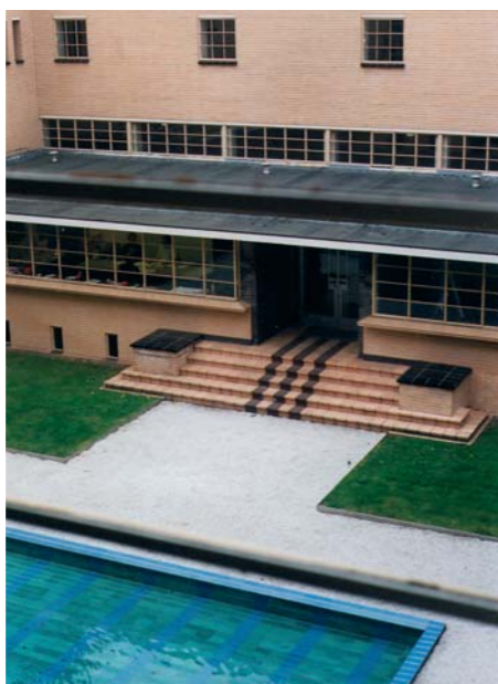
A 'red carpet' of dark quarry tile paving leads up to the main entrance defined by the roof which sweeps out in a cantilever, and the stepped side wall which becomes the balustrade wall.
