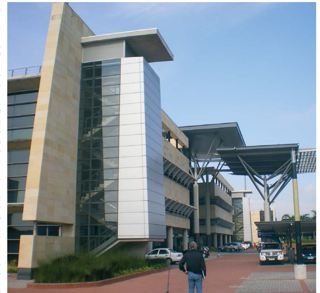
Standard Bank, Kingsmead Office Park, Durban. Elphick Proome Architects.
