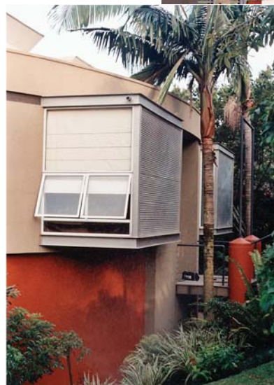
LEFT: Bedroom expansions to villa of 1991. To extend the children's bedrooms, right-angled bays of steel construction were cantilevered from the cylindrical form of the existing villa.
