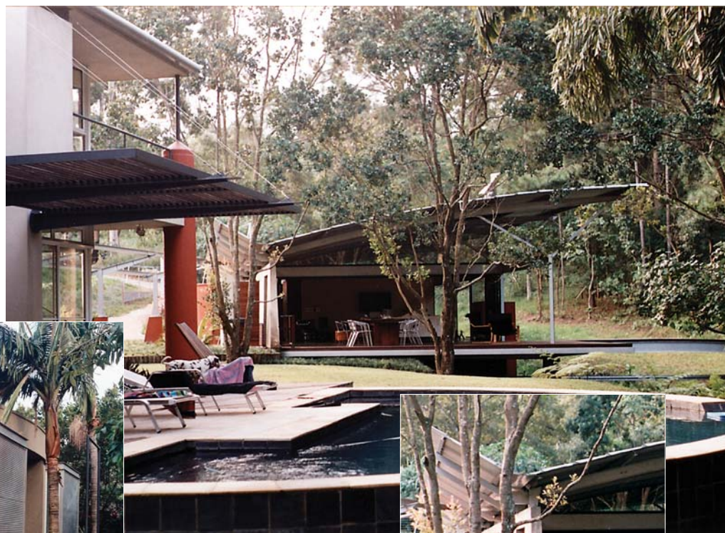
LEFT: Bedroom expansions to villa of 1991. To extend the children's bedrooms, right-angled bays of steel construction were cantilevered from the cylindrical form of the existing villa.
