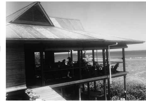
Detail of timber-framed structure with weather-board cladding.
