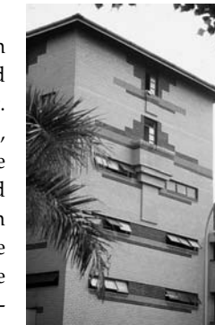
Thokoza Women's Hostel, Grey Street. Elevation to Dartnell Crescent.
