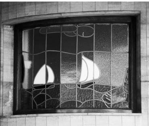
Coloured glass motif of sailing boats window in entrance foyer of Willern Court.
