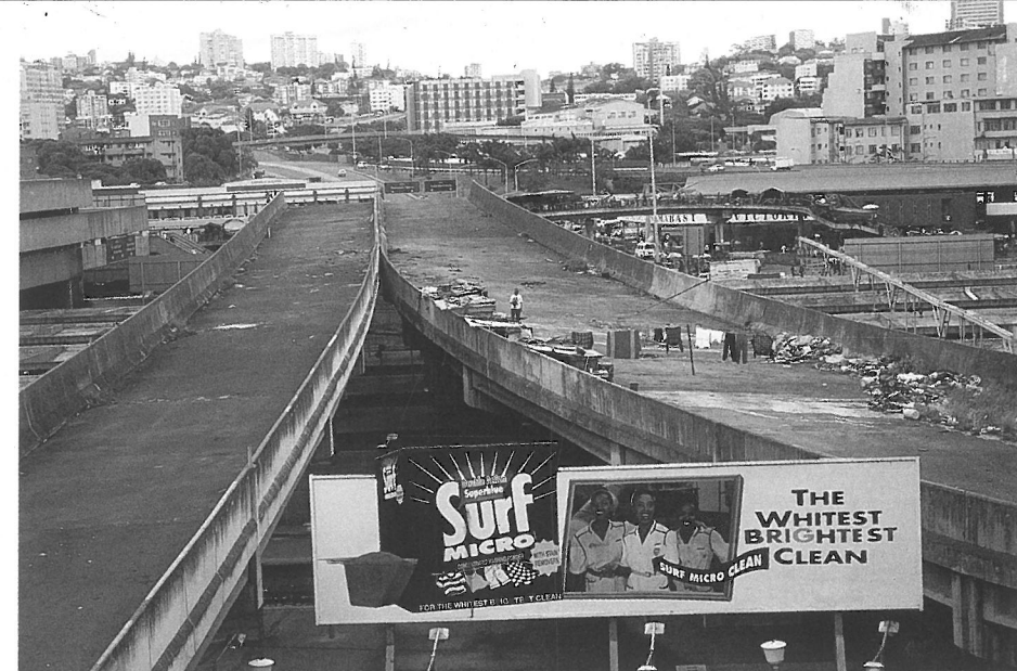
View towards Tollgate in west. Herb Traders Stalls – the site before...
