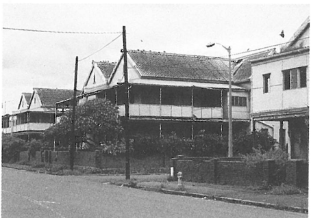
The enclave of semi-detached houses at Escombe Terrace, Point, deserted and decaying, 2001. Note the Bluff and the Millennium Tower under construction at left.
