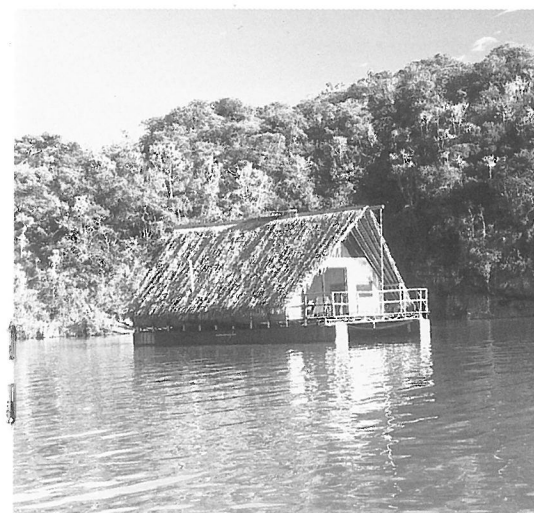
Chalets supported on pairs of fibreglass-clad polystyrene rafts and provided with underslung septic tanks.
