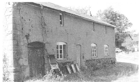
Blacksmith's shop before restoration
