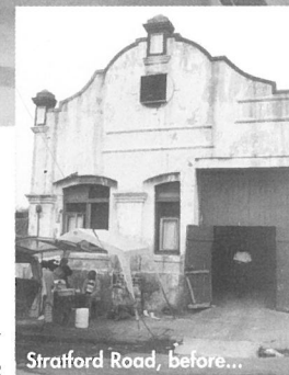
Stratford Road, before...
