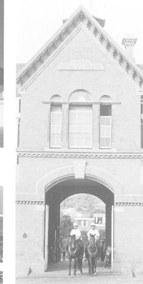
Alexandra Road Police Station, Pietermaritzburg
