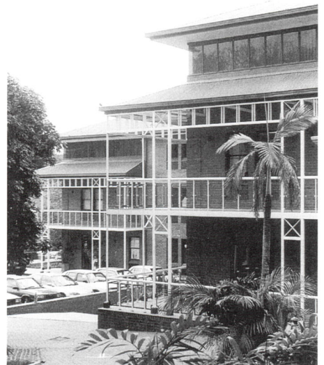
Atherton Office Development, 291 Florida Road, Durban Stafford Associate Architects cc
