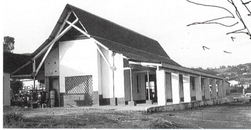
ABOVE & RIGHT: Dining hall LEFT: Children's Home
