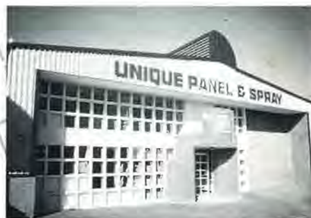
7. Unique Panel & Spray, 1990, Elphick Proome Architects
