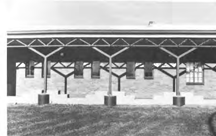
DETAIL OF WEST FACADE
