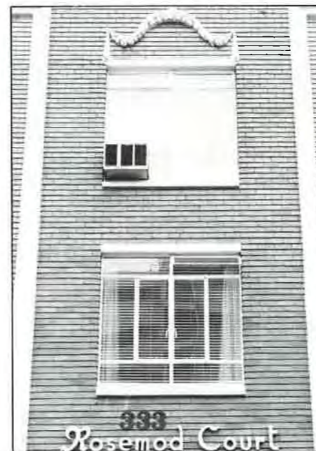
15 Rosemod Court, Musgrave Road, by Fritz Kass, stucco garland on functional modernist brickwork.
