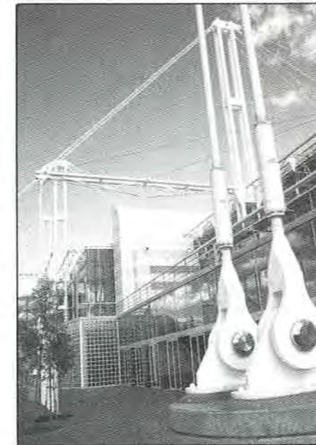
14 The new National Exhibition Centre at Darling Harbour, Sydney, by Philip Cox and Partners.
