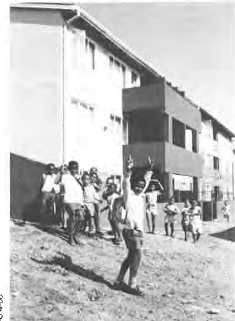
Balconies added to existing blocks of flats.
