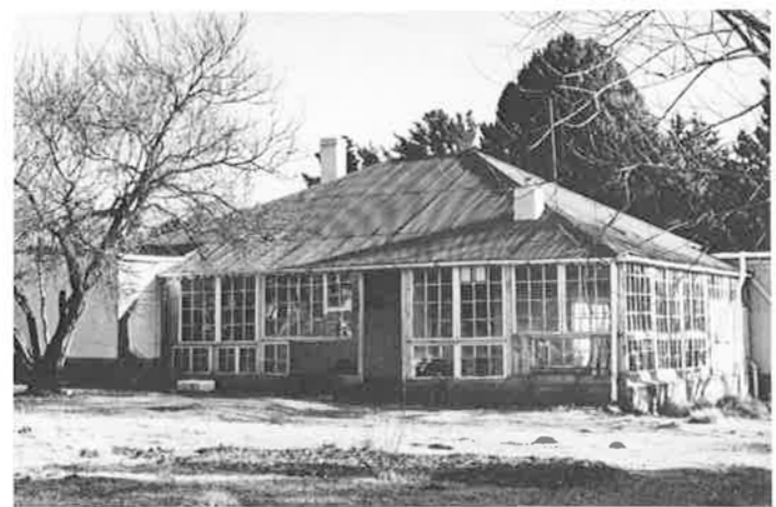
A north-facing verandah of an existing house, glazed to conserve warmth, a principle exploited in the Trombe wall.
