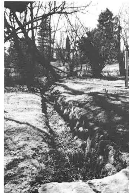
ABOVE: Vestiges of an old irrigation channel which drew water from the Bell River higher along its course.
