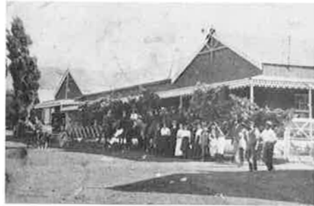
Rhodes Hotel, originally known as Horseshoe Hotel, built c.1898. Sited opposite the tennis courts — in the former Market Square — this building forms the heart of present day Rhodes.
