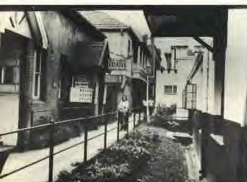
CHANGE LANE 231 LONGMARKET STREET. A tragic loss of Victorian porticoes. Before and after
