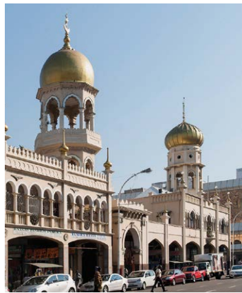
THE GREY STREET MASJID The original 1881 structure accommodated 48 worshippers. It is now one of the largest mosques in the Southern Hemisphere.
